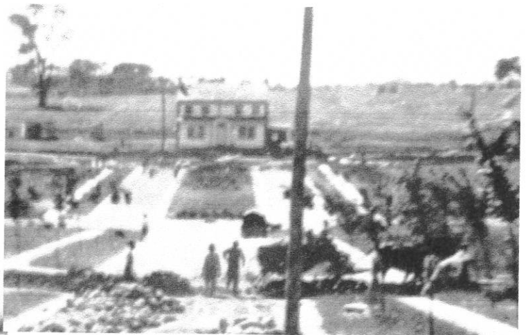
Construction of Schmelzer Island; North of Verkler Home
